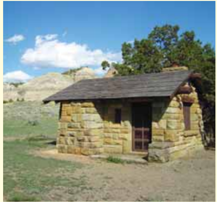
Old East Entrance Station, Theodore Roosevelt National Park (photo courtesy Mary Brazell, NPS)
